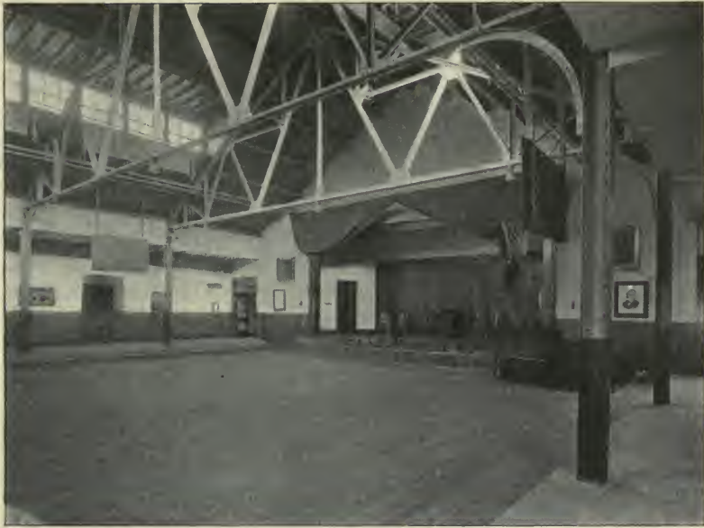
Assembly room and gymnasium
